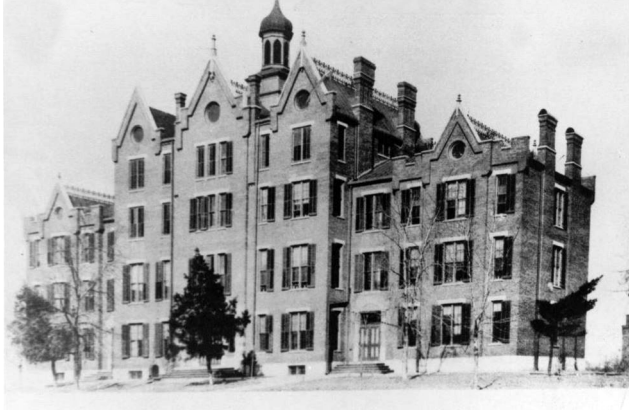
Figure 9. The Methodist English and German College, Quincy, Illinois, 1884. The building housed the college from 1847 to 1875, after which it was sold to the Quincy School Board and renamed the Jefferson School. At one time, two Nauvoo Temple capital sunstones were displayed on the school property. Quincy Area Historic Photograph Collection, Quincy Public Library, Quincy, IL.
