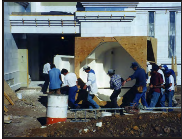
The font was carried into the temple before metal door frames were installed, December 22, 1998.
