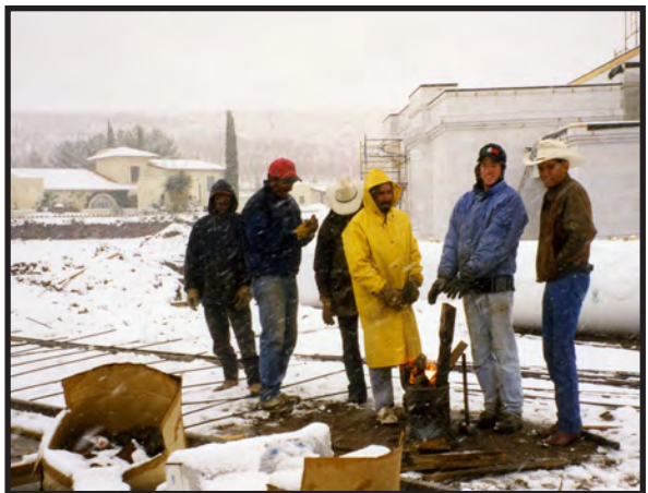
Concrete crew continues working despite blustery weather in early December.
