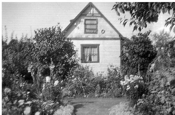
Fig. 10. The Zwick family acquired this small garden house just before the war and lived in it after they were bombed out. (F. Zwick)
