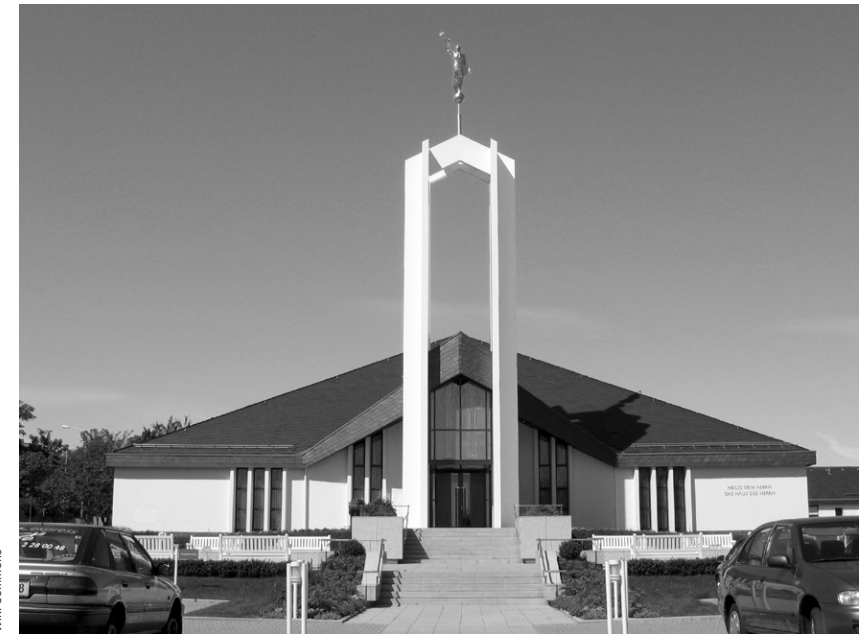
The construction of the Freiberg Germany Temple is one of the great miracles in the history of the Church in Europe. It is a wonderful example of how God can make the impossible possible in any part of the world.
