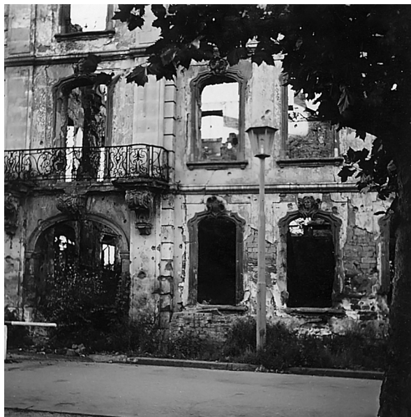
Fig. 9. The building on Kronprinzenstrasse where the Saarbrücken Branch had held its meetings was still a ruin a few years after the war. (H. Reger)
