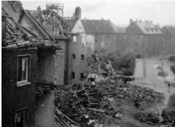
Fig. 9. Air-raid damage done to the apartment house in which the Schwiermanns lived. (A. H. Schwiermann)
