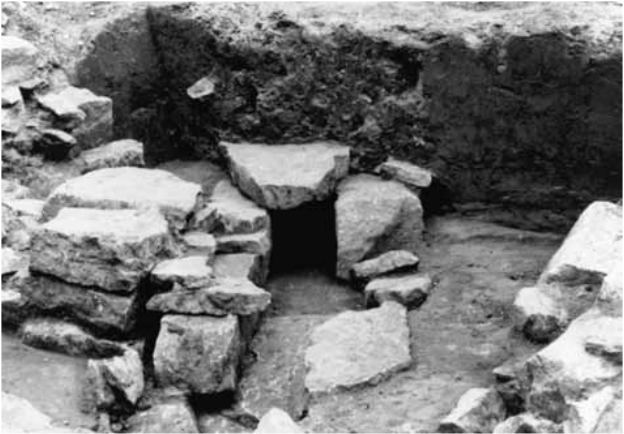
Figure 9.7 Font Drain, photograph, 1960s, LDS Church Archives. This photograph was taken facing southeast; the font drain has an opening of 12 inches square.
