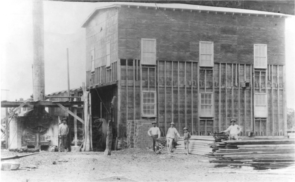
The Nuttall sawmill in 1899 as it was being dismantled to move it to Bryce. Note the shape of the burner on the left (which is usually tepee-shaped); potential spontaneous combustion of the sawdust made a burner imperative. Photo courtesy of Craig M. Reay.
