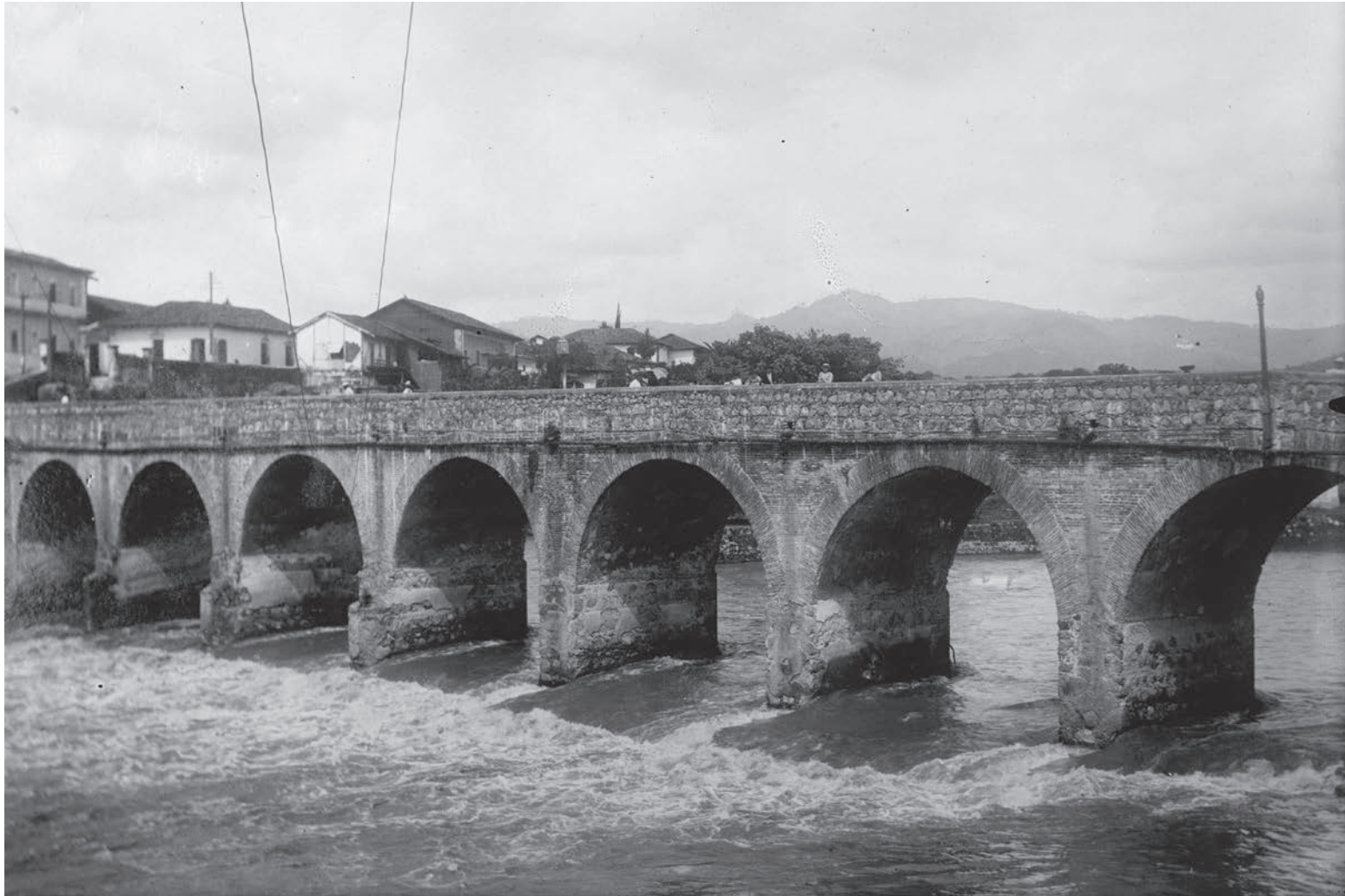
Bridge construction in Tegucigalpa, Honduras, ca. 1915. Library of Congress.
