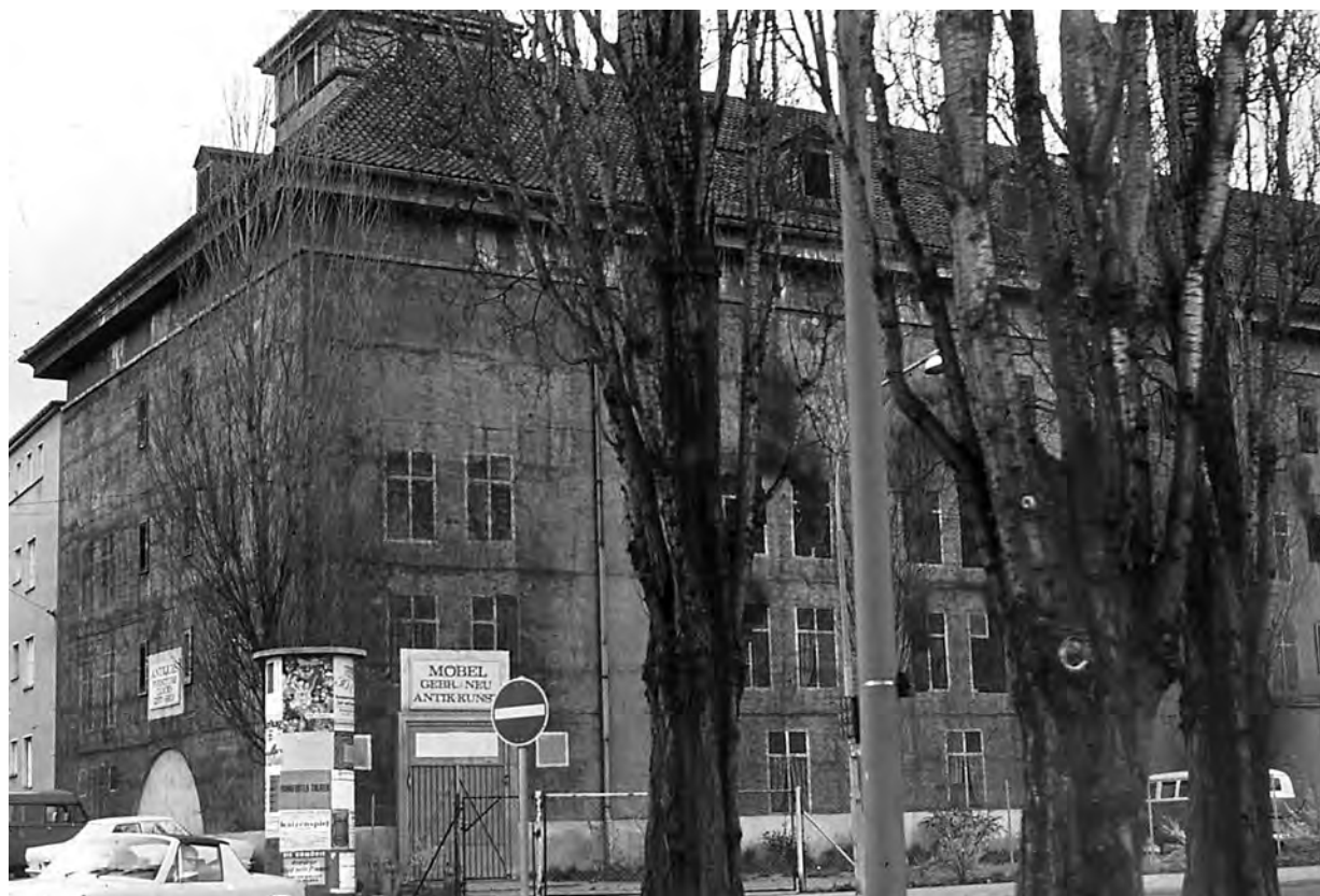
Fig. 9. This public air-raid shelter in northwestern Frankfurt was painted to represent an apartment house that had been attacked and was burning, apparently in an attempt to deceive enemy dive-bombers looking for targets. (R. Minert, 1973)
