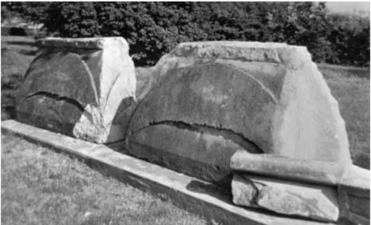
Figure 6.6 (Top) Sun Stone, photograph, date, and photographer unknown, LDS Church Archives. This sun stone was originally part of the Nauvoo temple. Known as a capital, it was composed of five stones that combined together weighed over 4,000 pounds. A sun stone was placed at the top of each pilaster shaft. One of the sun stones being reproduced for the reconstructed temple required 358 man-hours with the use of modern powered chisels.
