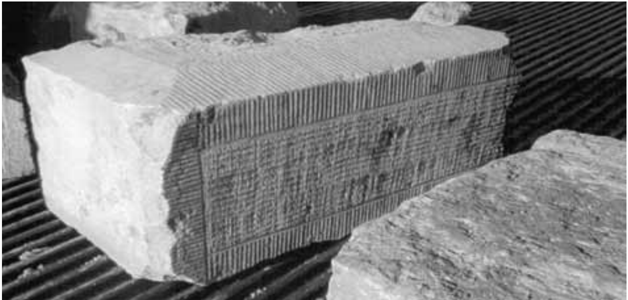
Figure 6.4 (Top) Stone with Vertical-Striation-Textured Finish, photograph, 7 April 2000, Ronald J. Prince, project manager, Nauvoo Temple Reconstruction Project, The Church of Jesus Christ of Latter-day Saints. This stone, typical of those used in main wall panels of the temple between pilasters, measured 8 inches in height by 23 inches in length. Buried for nearly 150 years, it was uncovered on 7 April 2000 as workers were clearing the site in preparation for rebuilding the temple. As a result of being covered and sheltered from the elements, it had been preserved in excellent condition. This stone had been given a vertical, striation-textured finish—sometimes referred to as an axe hammer strike—with fairly uniform vertical lines or grooves. Groove depth averaged no more than \frac{3}{32} of an inch and was generally spaced \frac{3}{8} of an inch from ridge to ridge on each side of the grooves.
