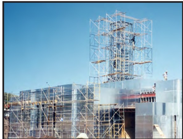
Aluminum-clad plywood forming the temple's exterior in September 1998.
