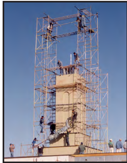
With no crane to assist them, workmen hoist the wrapped angel to the top of the temple's tower.
