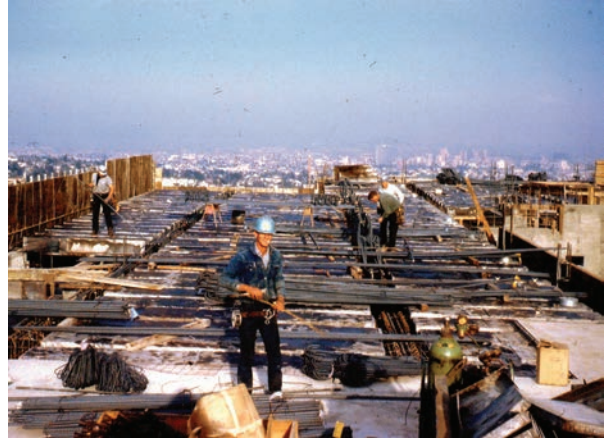
Top: Placing rebar for first-floor concrete slab. Courtesy of Virginia Loder.
