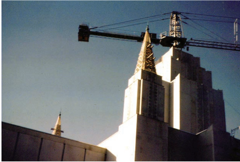
Work progresses on the small towers. Courtesy of Virginia Loder.
