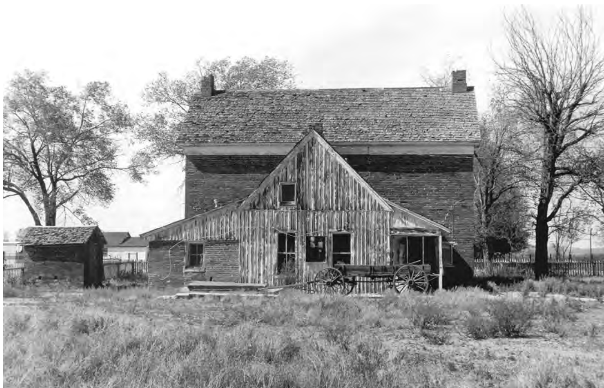
John Bushman built this frame house in Joseph City for his families and then later added the two-story brick home which is attached (see p. 91 for front of brick house). He fired his own bricks and made his own nails. Parked by the house is the ubiquitous covered wagon (sans cover); William E. Ferguson, photographer, about 2000. Photo courtesy of William and Betty Ferguson.
