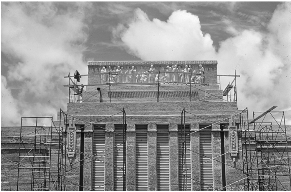
The friezes were hoisted into place and mounted around the cornice of the temple. Courtesy of Church History Library.
