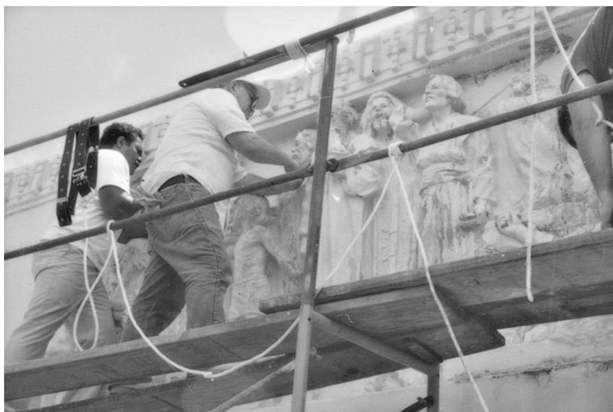
Removing layers of old paint during the 1987 restoration of the friezes, the craftsmen uncovered “a veiled masterpiece.” Courtesy of BYU–Hawaii Archives.
