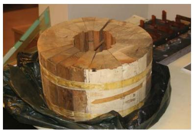
Cross section model of a gallery column. The pillars that hold up the gallery were constructed from wood but made to look like stone. Tall sections of pine were cut into wedges and bound together, forming a straight, hollow pillar. The columns were then sanded and painted to resemble fine marble. *Courtesy of Richard Crookston*
