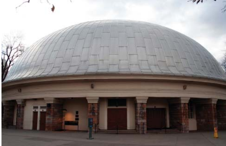
Over time, the Tabernacle roof has had several surfaces, including wood and metal, such as the aluminum roof shown above, which was installed in 1947. Courtesy of Richard Crookston
