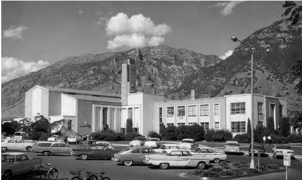
The original Joseph Smith Building. Designed by Fred L. Markham, the building stood for fifty years, from 1941 to 1991. Its replacement was designed by his two sons, John and Dix (see page 61). Courtesy of L. Tom Perry Special Collections, Harold B. Lee Library, BYU.
