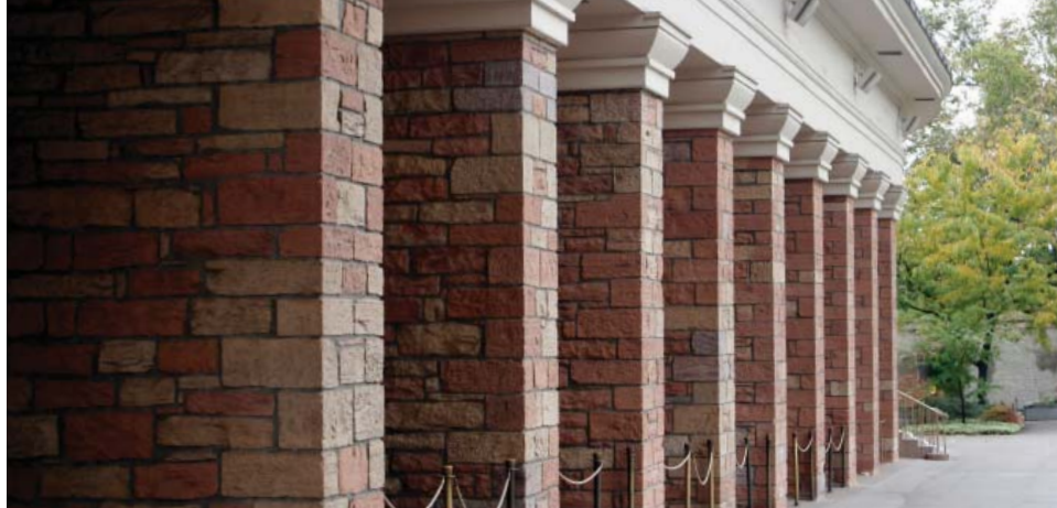
The Tabernacle roof is supported by forty-four stone piers built of red sandstone (see pages 151–52). Courtesy of Richard Crookston
